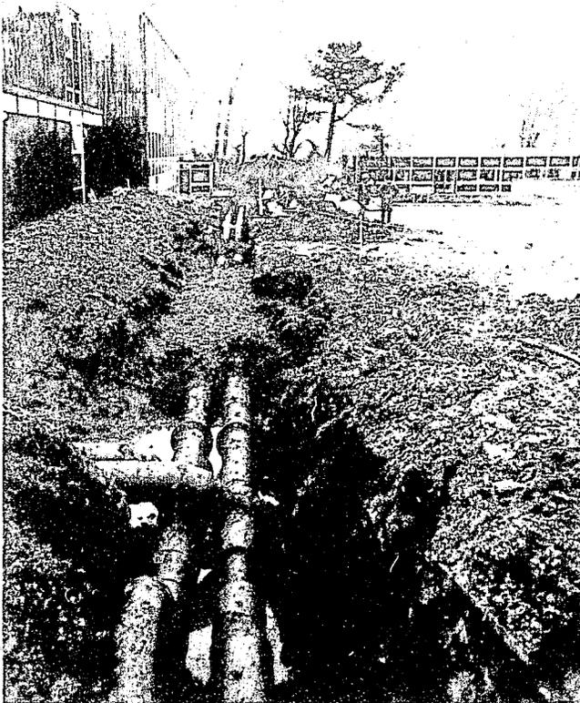
Earthworks at headquarters during the installation of a new heating system.
