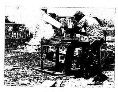
Inmate using masonary saw to shape concrete blocks to the correct size at Walton C.I.
