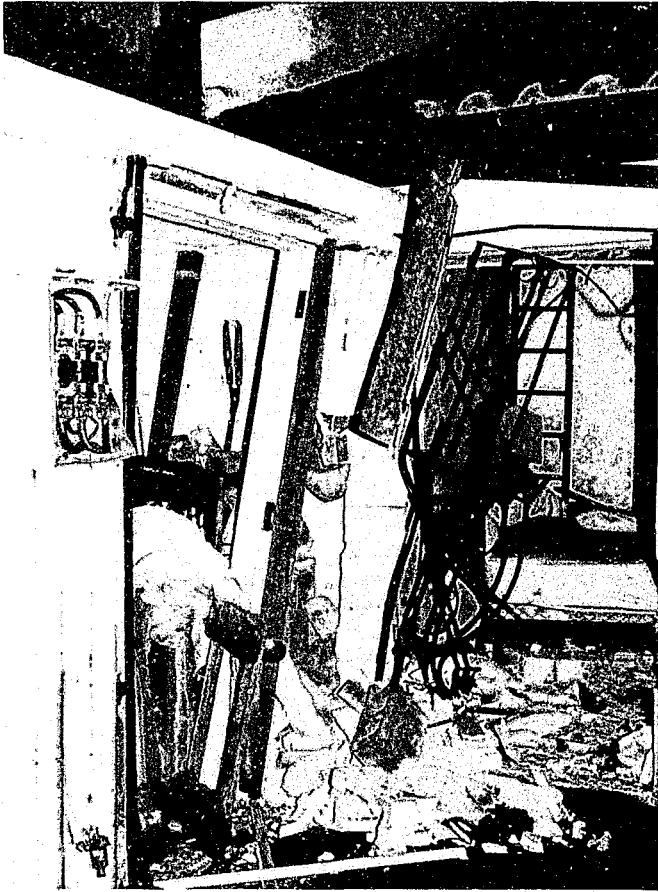
Damage to a residence caused by a pipe bombing that occurred on November 29, 1991.
