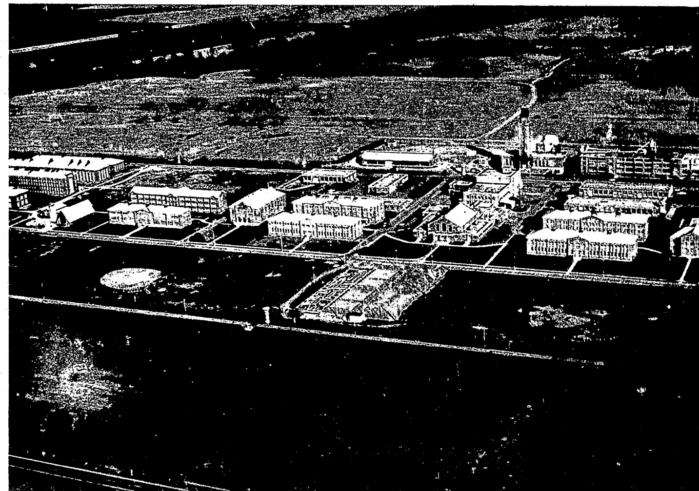
The Chillicothe Correctional Institute, just north of Chillicothe in Ross County, was formerly a federal reformatory. It opened as such in 1925 and was leased by Ohio in 1966. A 1500-acre self-contained community, the main institution consists of a 72-acre compound of more than 50 buildings. The facility includes a 962-acre farm operated by residents. The institution also serves as a reception and classification center for offenders over the age of 30 and those under 30 with prior felony convictions. Operated as a part of the institution is Hocking Honor Camp in Hocking County. The staff of the facility totals about 500; residents number approximately 1200. Operating expenses for fiscal year 1973 were $6 million.
