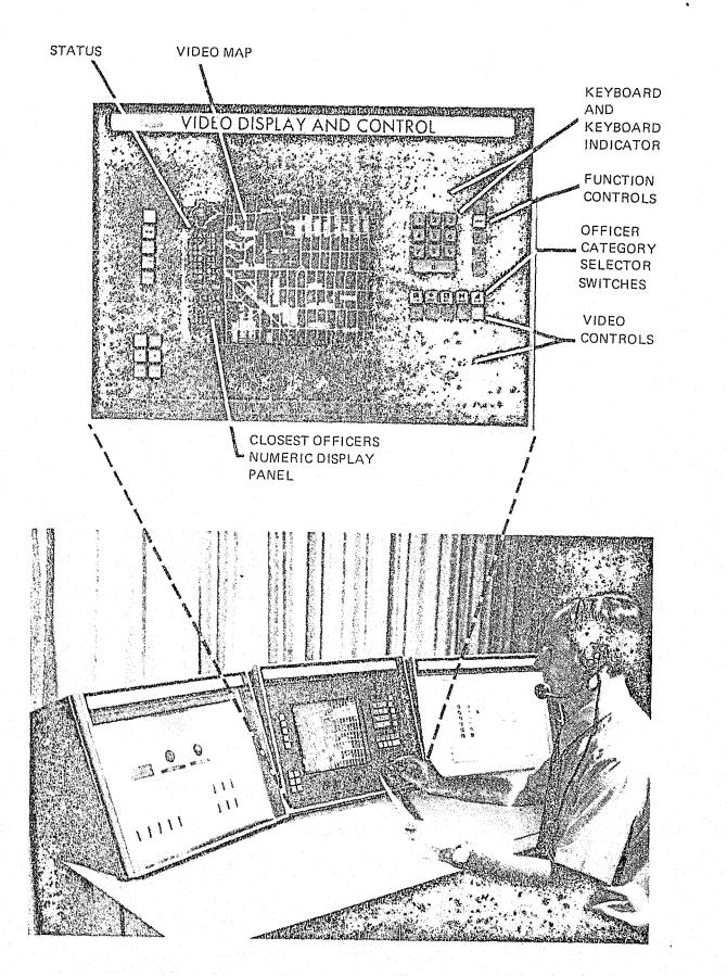
FIGURE 2 - VIDEO DISPLAY AND CONTROLS
