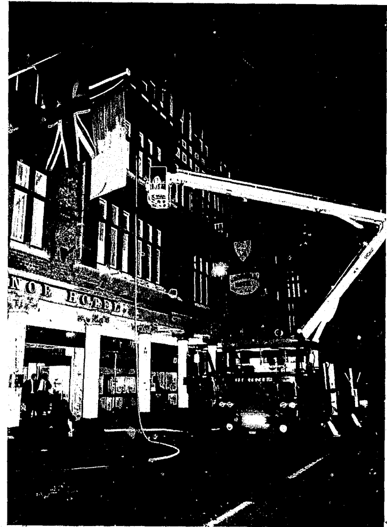
During the evening of Tuesday, 14th August 1973, a fire was discovered at the Grosvenor Hotel, Eastgate Street, Chester, and damage to the structure and interior fittings amounting to approximately £100,000 was caused. This was the largest fire in the city for 16 years and fortunately there were no persons injured.
