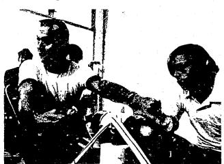
Demonstration of the filling of air bottles to be used in diving.
