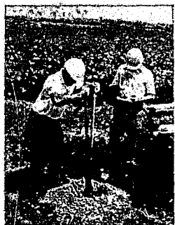
Digging the hole.
