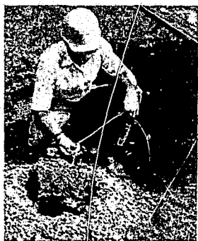
Inserting the detonating cord.
