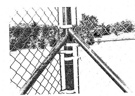
Figure 155. Fencing Using American Fittings To Attach Tensions Bars to Poles
