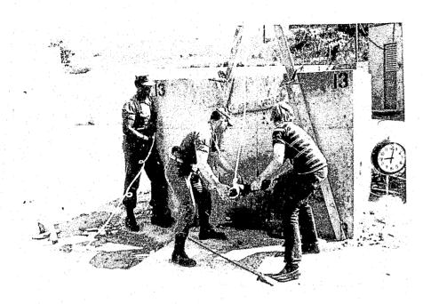
Figure 123. Test 13K. Two-man Operation of Suspended Battering Ram
