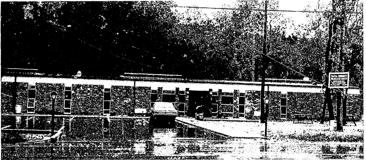
A recently constructed, 60-man pre-release center in Charleston, South Carolina. Photo by Andy Habingreither.
