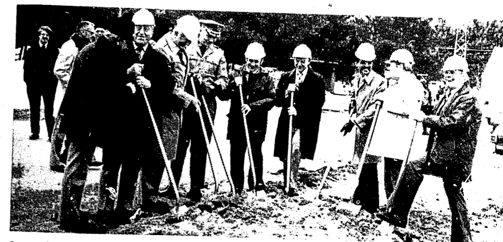
Groundbreaking signals the start of construction of a $3.8 million State Police facility at Ray Brook at which security for the 1980 Olympics will be coordinated. At left, facing camera, is the late Ronald MacKenzie, president of the Lake Placid Olympic Organizing Committee, who died at year's end. Next to him are Superintendent Connelie and Asst. Dep. Supt. Jerome J. McNulty, head of the Uniform Force, followed by Tom Monroe, regional director of ENCON; Mayor Robert Peacock of Lake Placid, Frank Jasmine, Governor's program associate; John Egan of the Office of General Services, and Rev. J. Bernard Fell of the Olympic committee.
