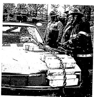
Proper method is practised in using hydraulic equipment to lift and pull steering wheel away from trapped victim.
