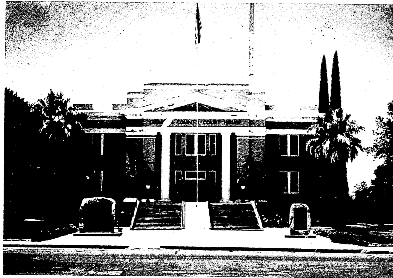
GRAHAM COUNTY COURTHOUSE
