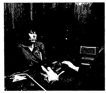
One new aid for investigators is the Psychological Stress Evaluator (P.S.E.) which the Department began using in January of 1981. The P.S.E. is a tape recording and charting device which enables a trained operator to determine voice stress in answers given to yes or no questions. The device actually enables the operator to measure the severity of voice stress exhibited by the subject.
