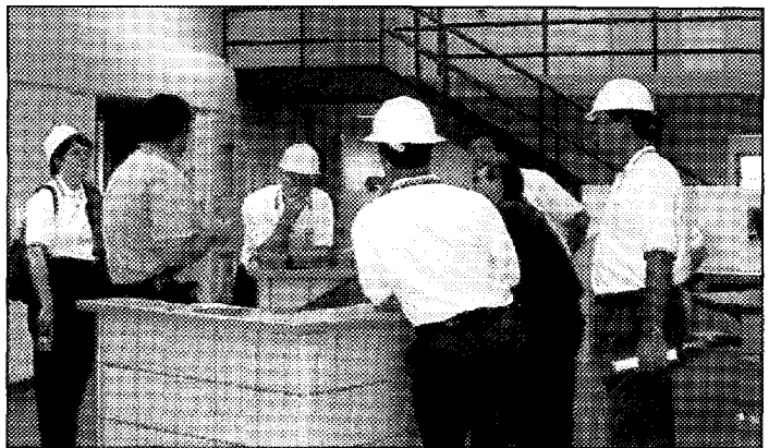
Above and bottom left: Institute participants tour an under-construction adult detention facility in Fairfax County, Va.
